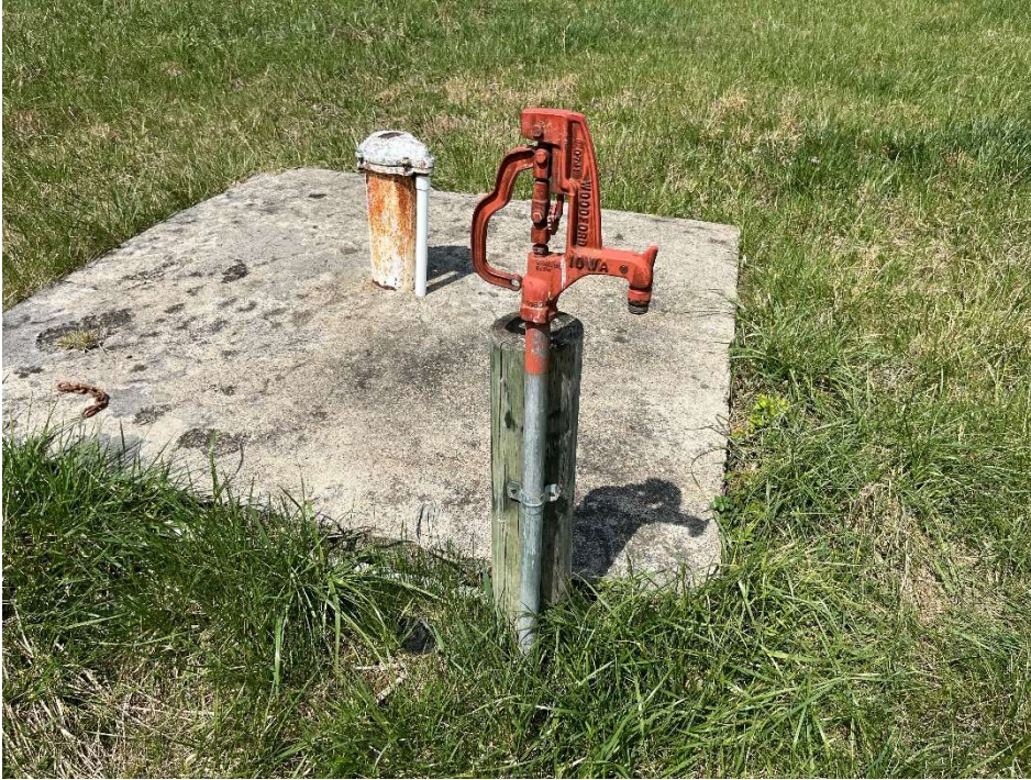
Figure 89: Close up view of the monitoring well.
