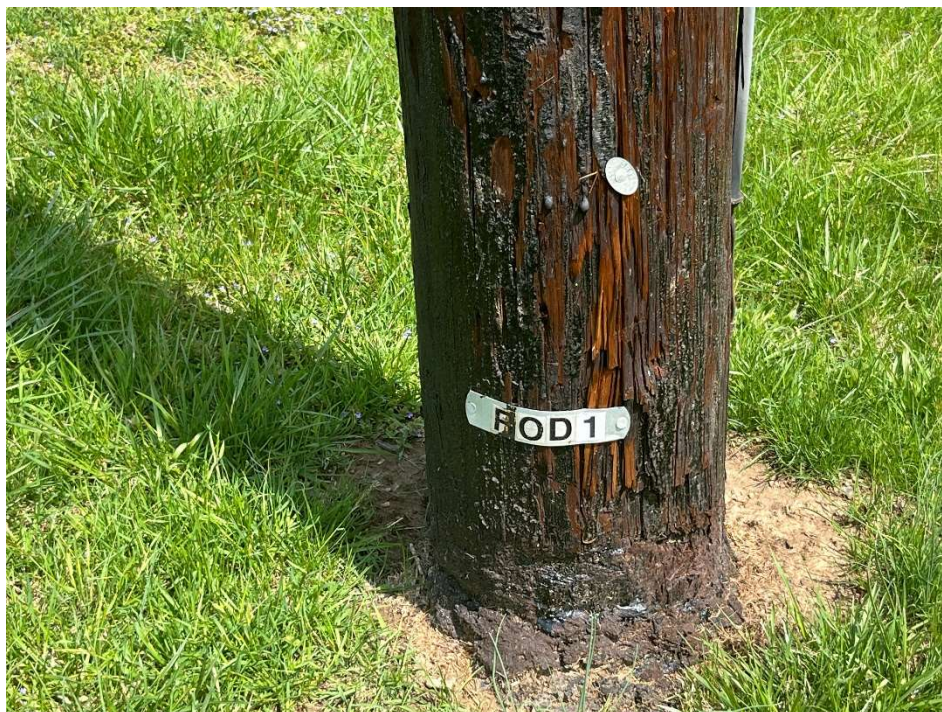
Figure 42: View of the bottom of the electrical pole.
