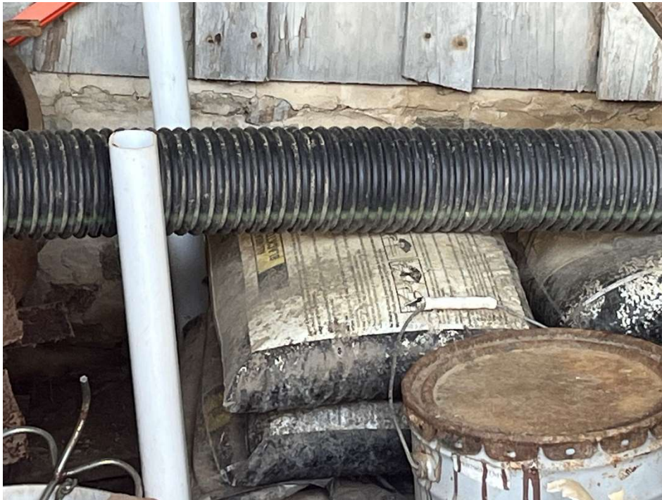
Figure 66: Close up view of asphalt repair bags.
