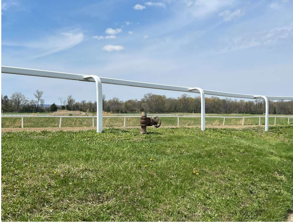
Figure 79: View of the old water sprinkler system spigot.
