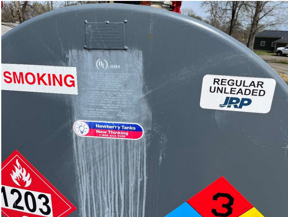
Figure 110: View of signage on the on-site fuel tanks.
