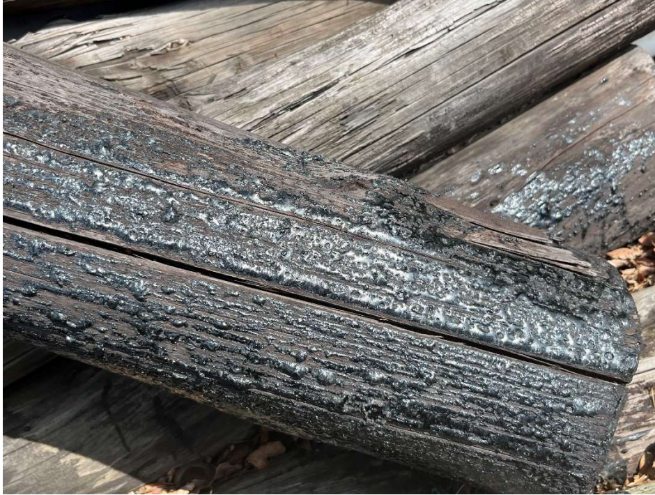
Figure 73: Close up view of the black substance on the ends of the poles.
