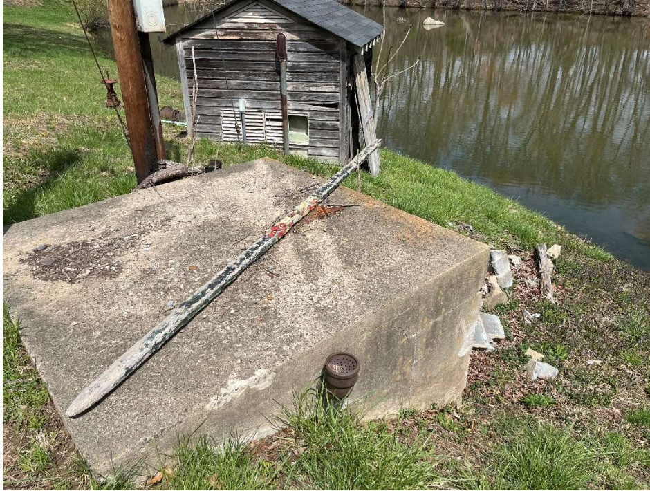
Figure 43: View of the old and new pump house by the onsite pond.
