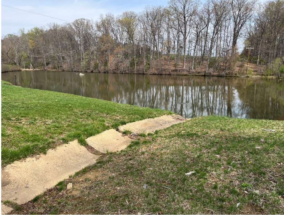
Figure 39: View of drainage channel that runs into the onsite pond.
