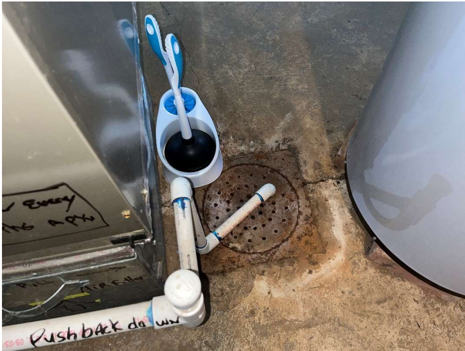
Figure 106: View of the drainage area in the basement for the one site residence.
