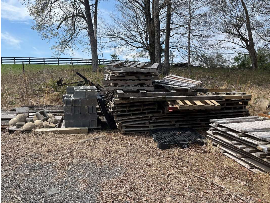
Figure 57: View of piled materials in trash area.
