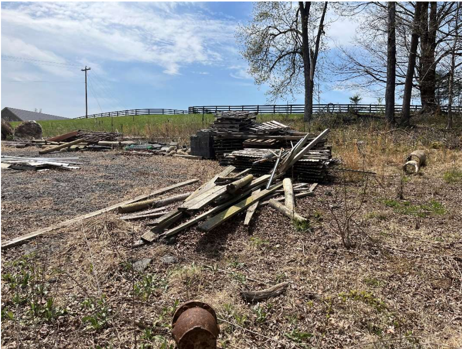
Figure 54: View of 2/2 staging areas on site where materials are stored on the northern side of the site.
