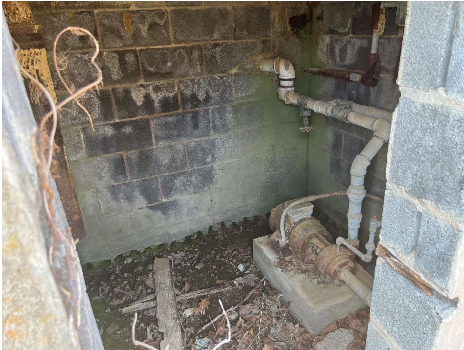
Figure 48: View of inside the old pump house.
