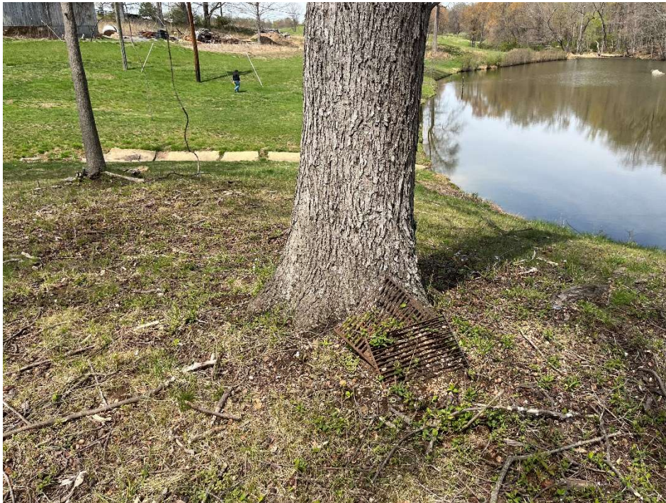
Figure 38: View of rusted metal located around the tree base by the onsite pond.
