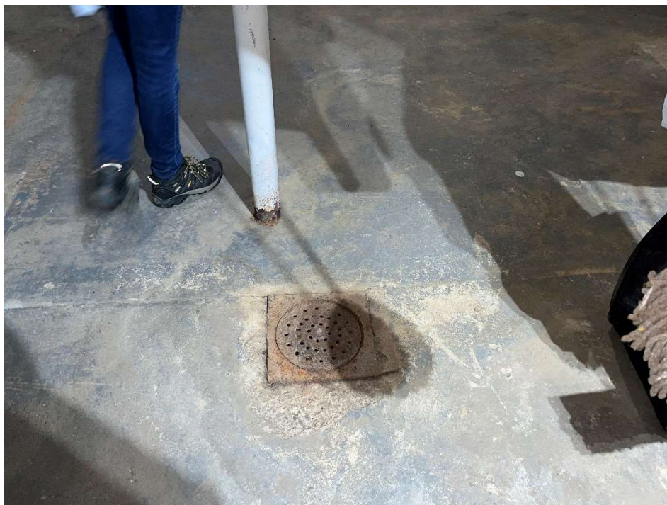
Figure 104: View of drain in the basement of the on-site residences.
