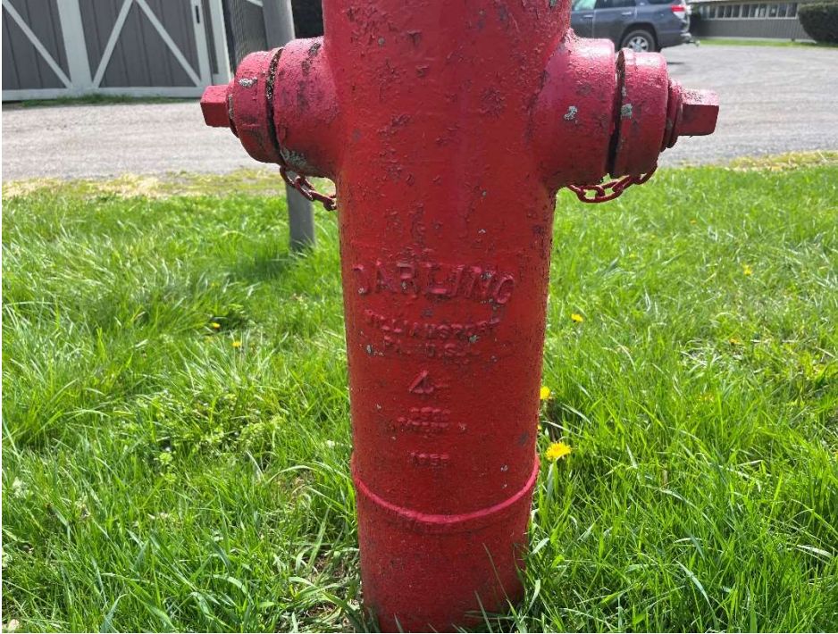
Figure 99: View of the back of the fire hydrant.
