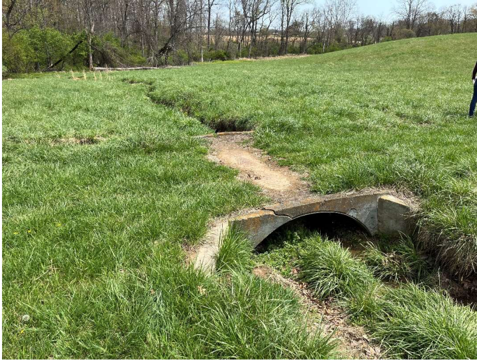
Figure 5: View of culvert on eastern portion of site.
