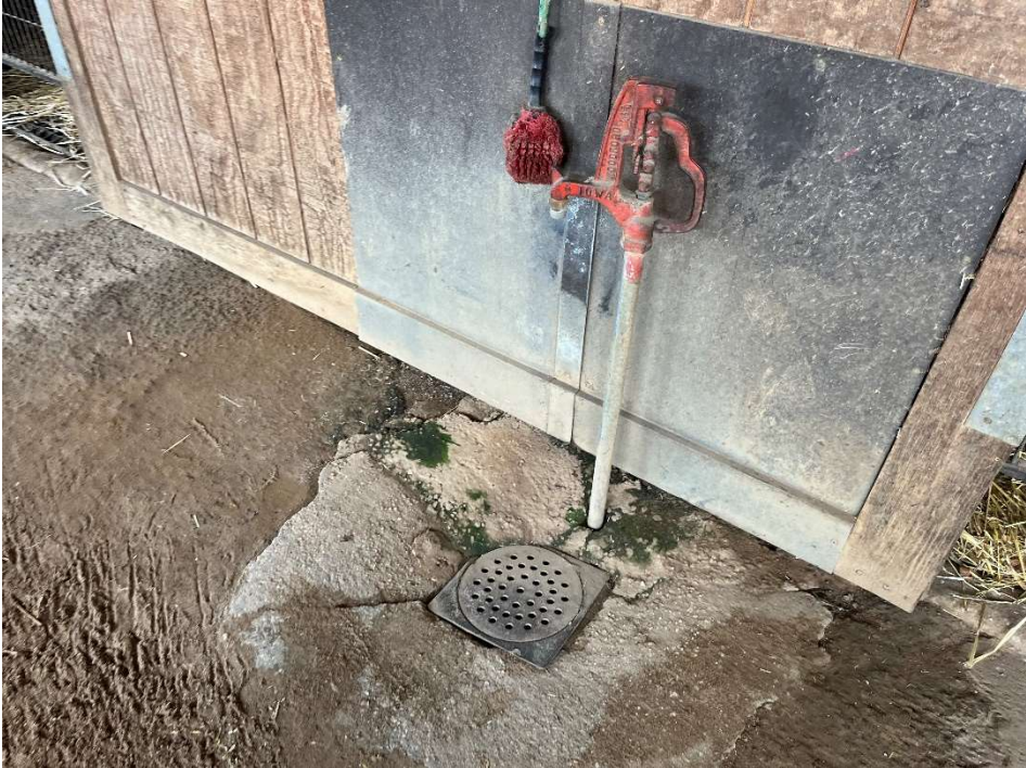
Figure 81: View of a water pump and drainage inside one of the barns.
